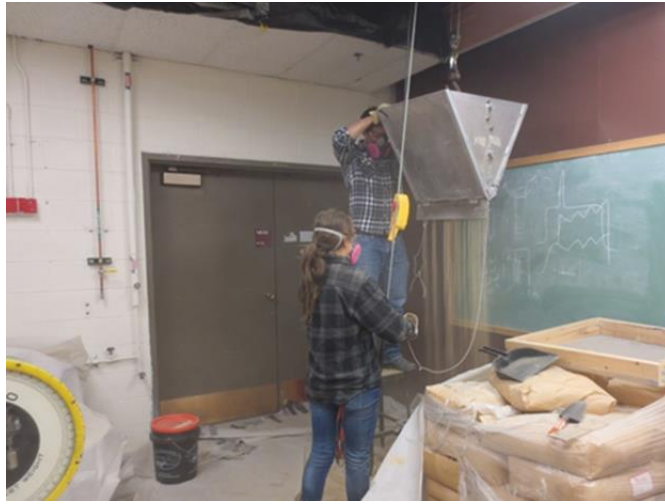
Figure 2.8. Soil model preparation by pluviation through a hopper.
