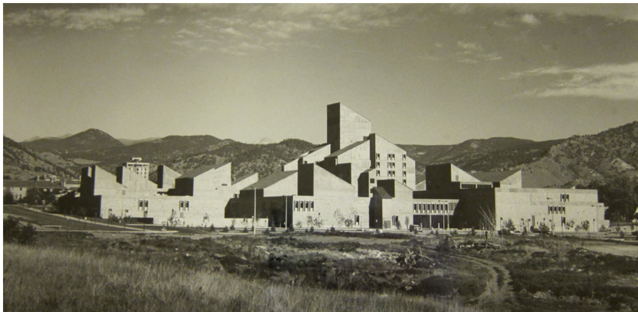
Figure 25: Engineering Sciences Center, 1966
