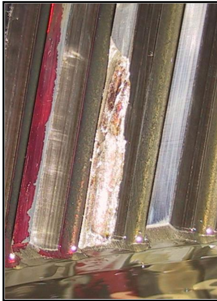
Figure 93: Gear tooth failure from an operational wind turbine, taken from [82]
