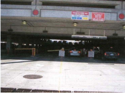
Photo # 1: Floyd Street Parking Garage
