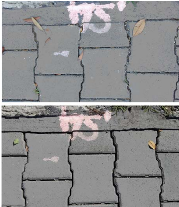
Figure 5: Visuals of practice 19 G before (above) and after (below) the maintenance
