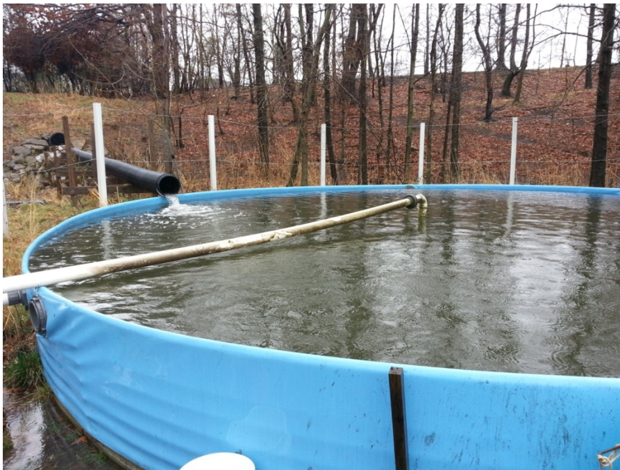
Figure 17: Primary tank for collecting stormwater runoff
