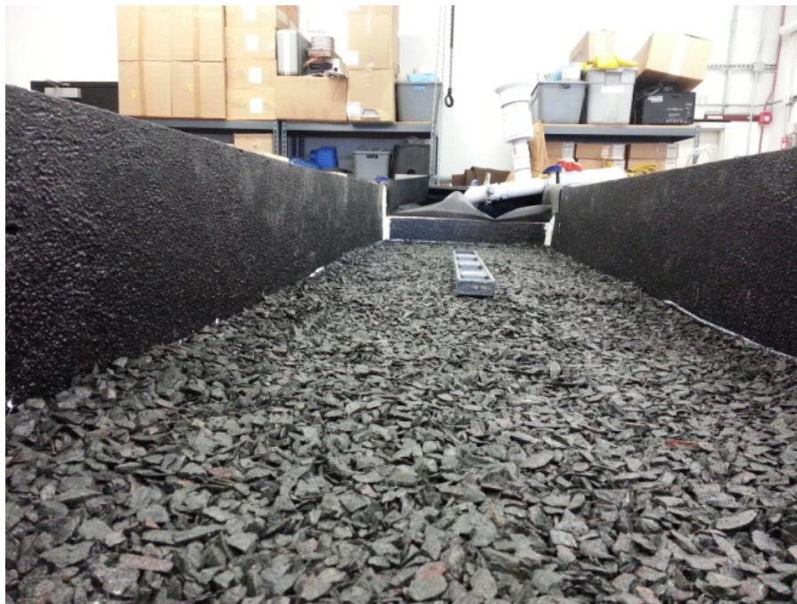
Figure 24: Compacted and leveled bedding layer
