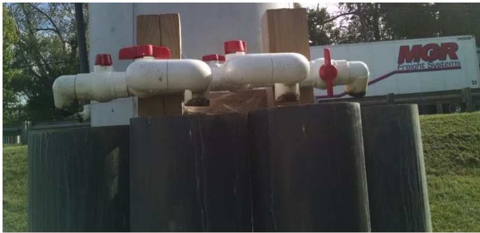
Figure 3.4 Inflow Control into Filters
