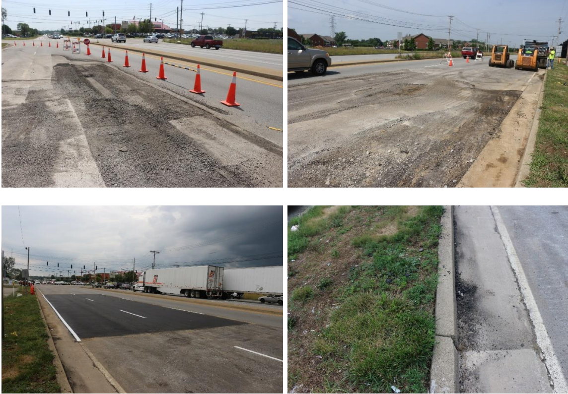
Fig. 5.2. Field view of utility cut restoration on Fern Valley Road in Louisville, KY
