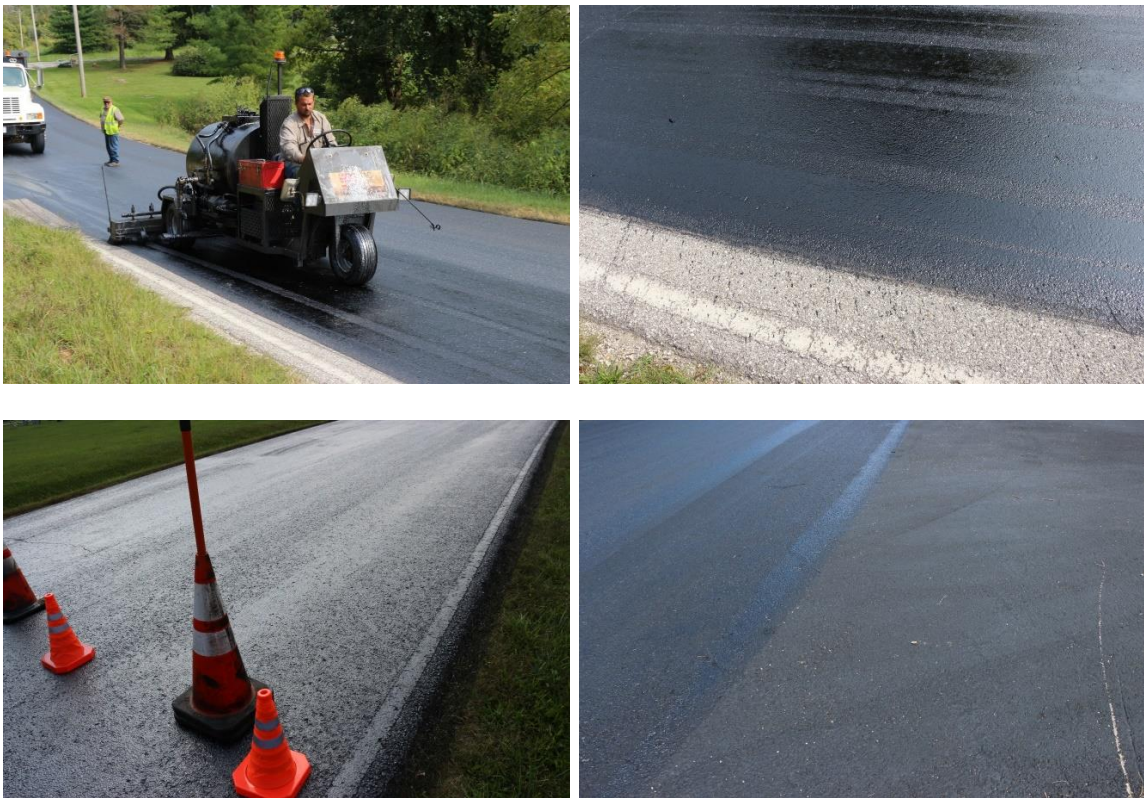
Fig. 5.1. Field view of rejuvenation on Heidelberg Road in Corydon, IN
