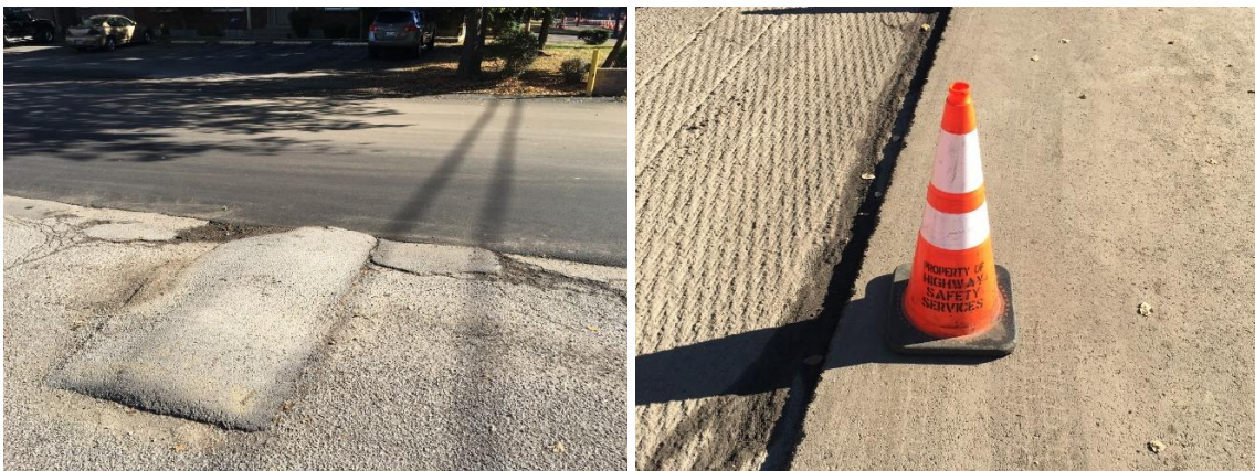
Fig. 5.9. Field view of mill and overlay on Craft Drive and Quest Drive in Louisville, KY
