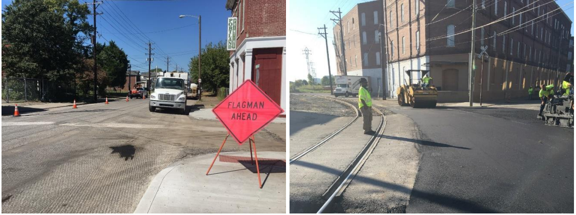
Fig. 5.8. Field view of mill and overlay on Portland Avenue in Louisville, KY
