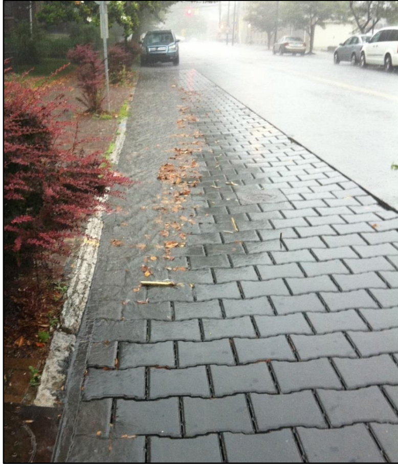
Figure 46 - Runoff Flow during a Rain Event, Control 19G
