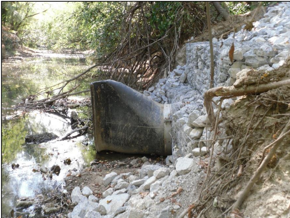
Figure 9 - Discharge Point of CSO130 to Beargrass Creek (Badwaterjournal.com 2010)
