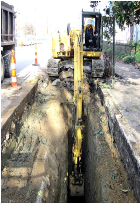
Figure 8. (a) Permeable pavement cross section schematic of controls 19G and 19H (b) Storage excavation of control 19G
