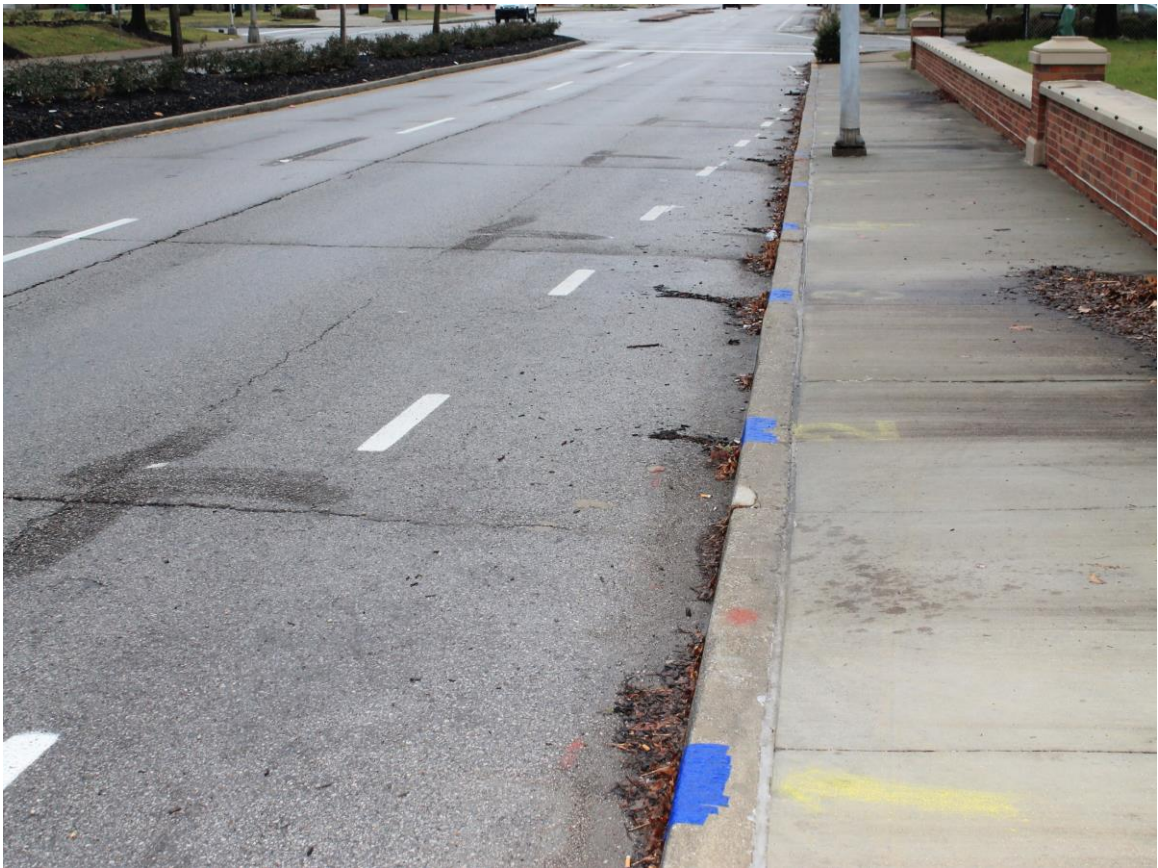
Figure 35: Method for the First Survey of the Newly-Developed Countermeasure for Bicyclists Safety-Turning Position
