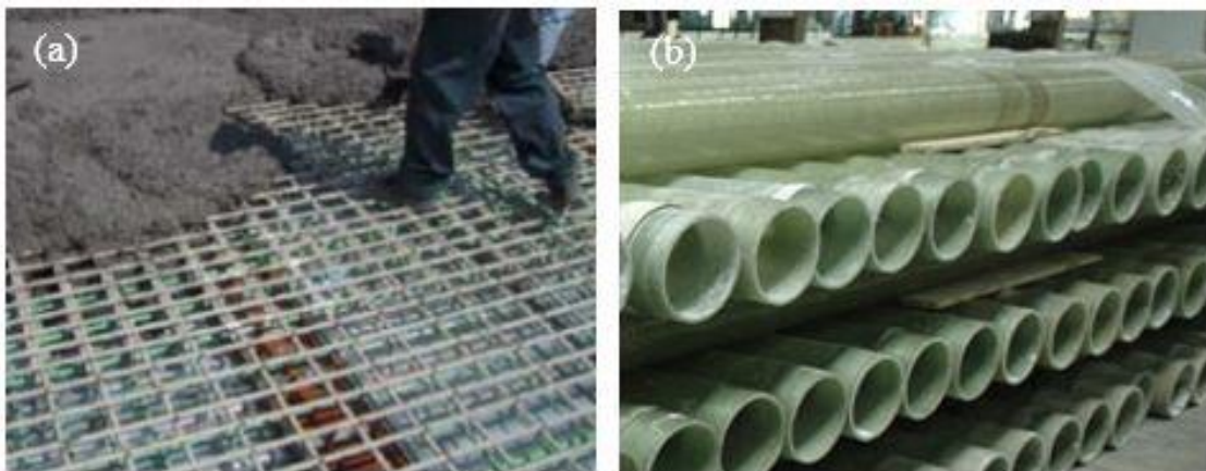
FIGURE 1 – FRP Structural Elements: (a) GFRP Bridge Decking (b) FRP Utility Poles
