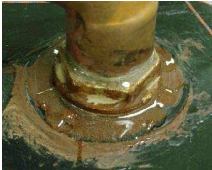
Figure 2.8 – Sealed heat pipe and water tank joint
