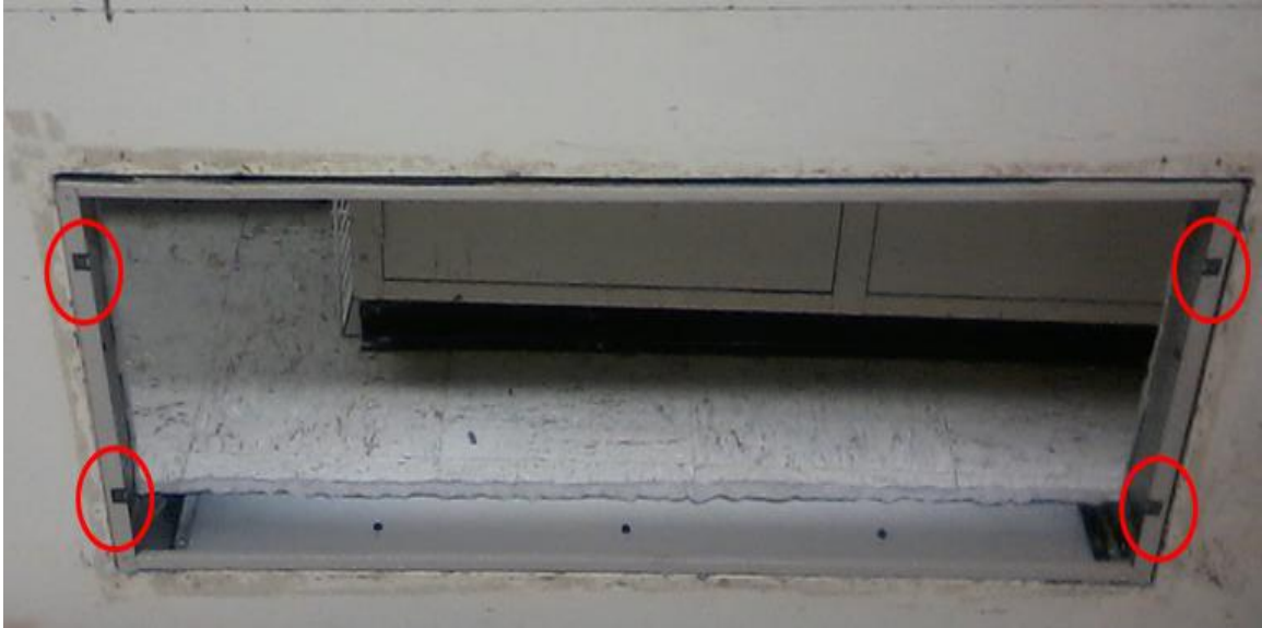
Figure 4. Mounting locations on the filler wall.
