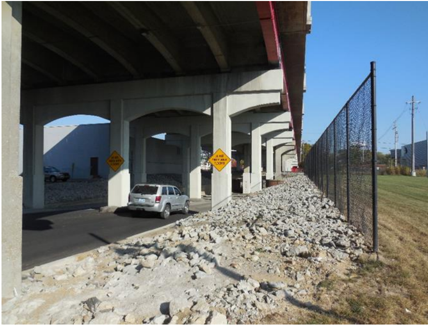
Figure 5. University of Louisville Belknap Railroad underpass.
