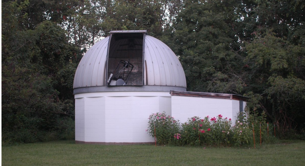
Figure 14. Outside view of MORC telescope enclosure. The enclosure is a dodecagon-shaped concrete block building with a rectangular control room on one side. An Ash-Dome brand dome sits on top of the block walls. The upper and lower shutters are raised and the MORC telescope is visible inside.
