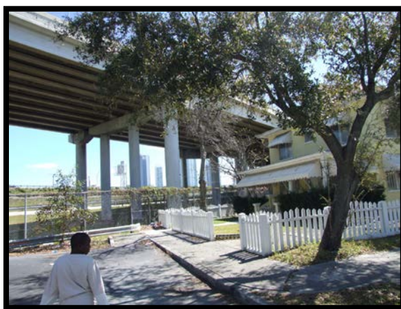
Figure 11 - Chapman House, built in the 1920s, is perhaps the most elaborate residence remaining today in Overtown however today is fenced in by the adjacent massive expressway ramps of I-95 and SR-836. Much of the surrounding area is vacant or deteriorated. Photo by author.
