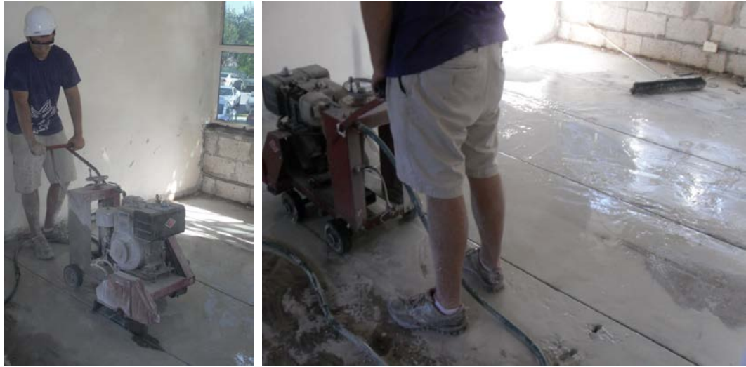
Figure A.32 – Saw-cutting of slab strips 1 and 2
