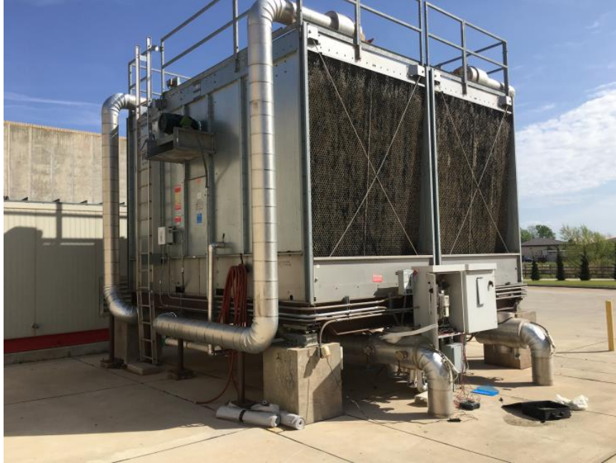
Figure 4-16 - VFD experiment facility.
