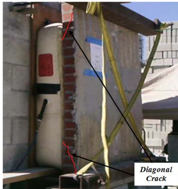
(f) (Enhanced crack lines)
