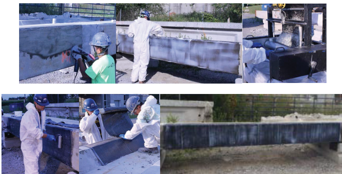
Figure 53 – FRP Application to Damaged PC Girder C
