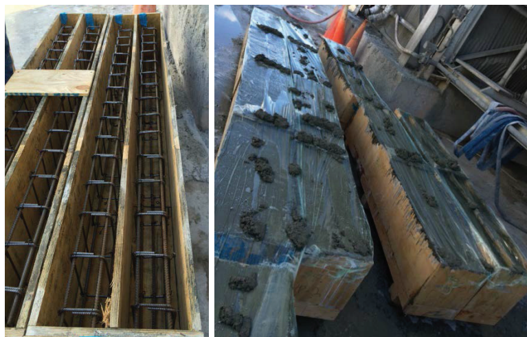
Figure 74 – RC Beam Formwork Prior to and After Specimen Preparation
