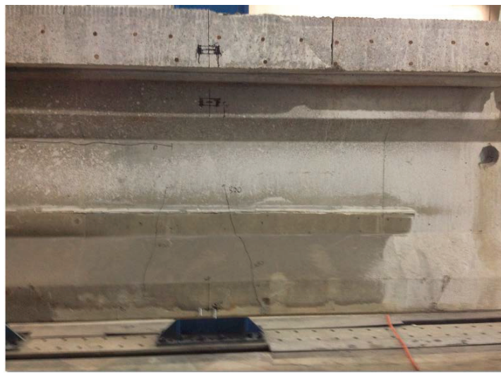
Figure 59 – Test A-1, Iteration 2 Flexural Cracks in the Bottom Bulb
