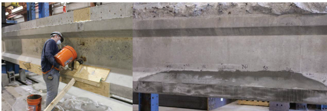
Figure 46 – a) Concrete Repair Formwork b) Repaired Area
