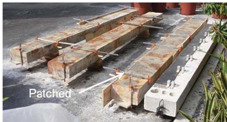
Figure 4.17 - Concrete patching chipped areas (B1 to B3)
