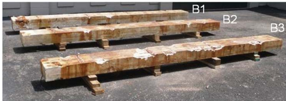
Figure 4.15 - Local removal of concrete cover (B1 to B3)
