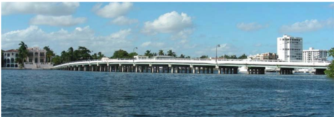
Figure 2.2 - Fair Isle Bridge from South-East direction
