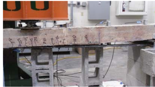
(b) Delamination B2
