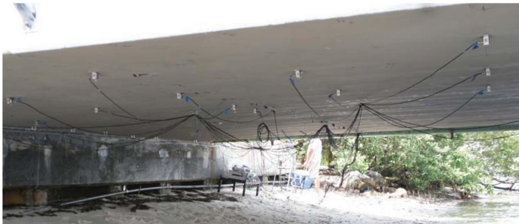
Figure 3.19 - AE sensors and strain gauges on the deck soffit
