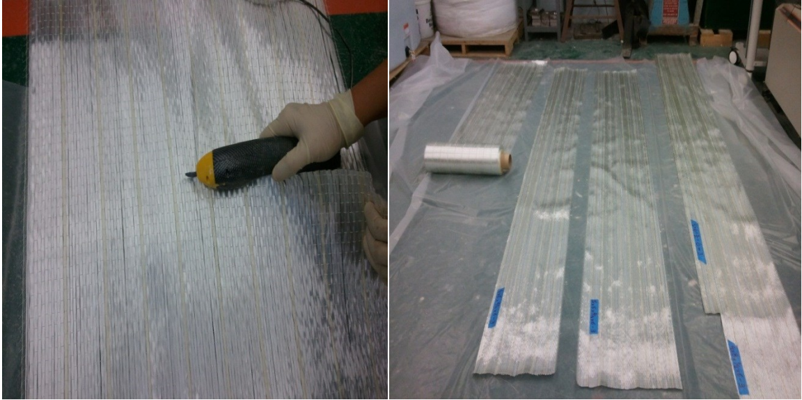
Fig. C-2: Cutting glass fiber sheets
