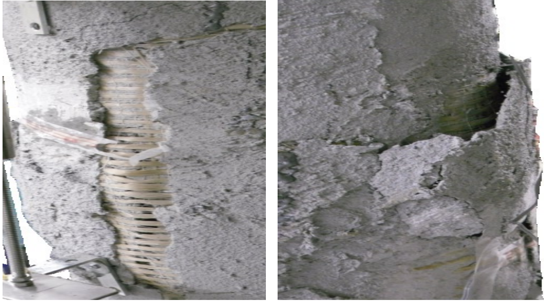
Fig. 4-4: Typical column element after testing
