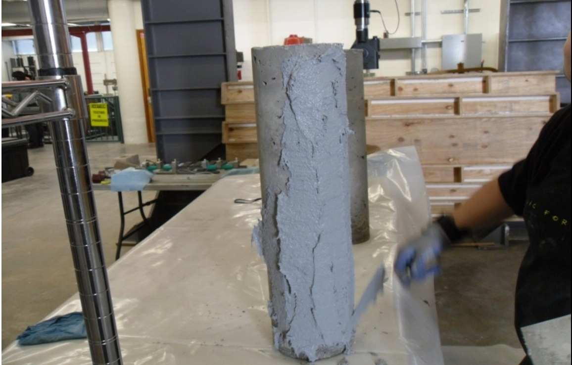
Fig. B-6: Application of the inorganic cementitious matrix
