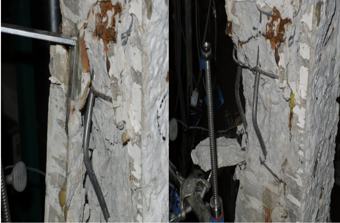
Fig. 3-4: Sample of failed control RC columns
