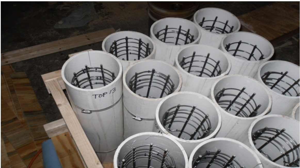
Fig. B-3: Reinforcement bars placed inside formwork
