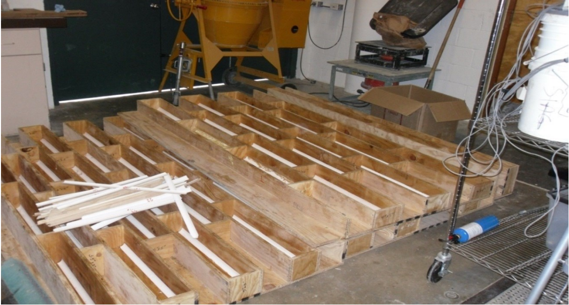
Fig. B-2: Formwork
