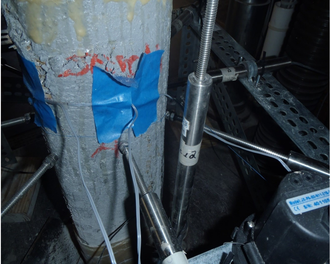
Fig. B-12: Failed PBO-FRCM wrapped circular column
