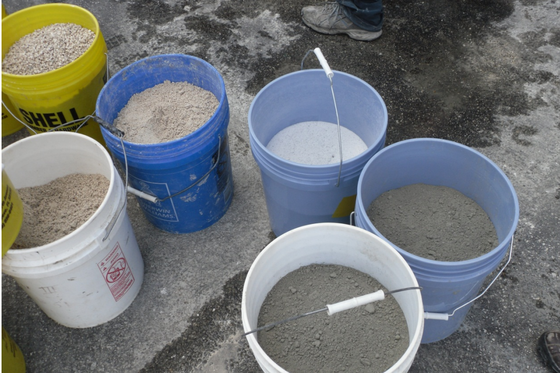
Figure B-2 - Materials for concrete mixing
