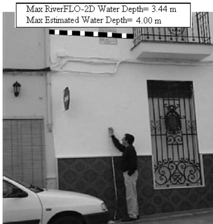
Figure 94. Sumacarcel Flooding Test. Water elevation mark and numerical water surface depth for gauge 10 in Jucar Street of Sumacarcel.
