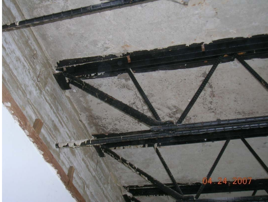
Figure 37 – Test Site: Open-Web Joist Support
