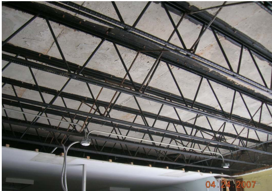
Figure 36 – Test Site: Open-Web Joists
