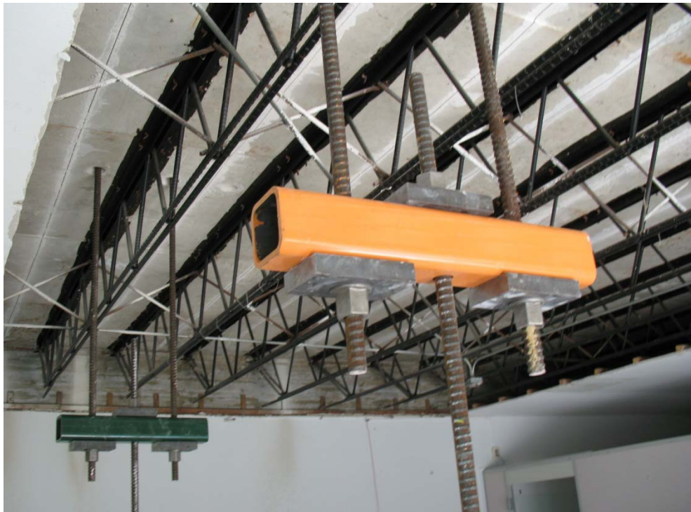
Figure 53 – Loading Setup (1 st Floor)
