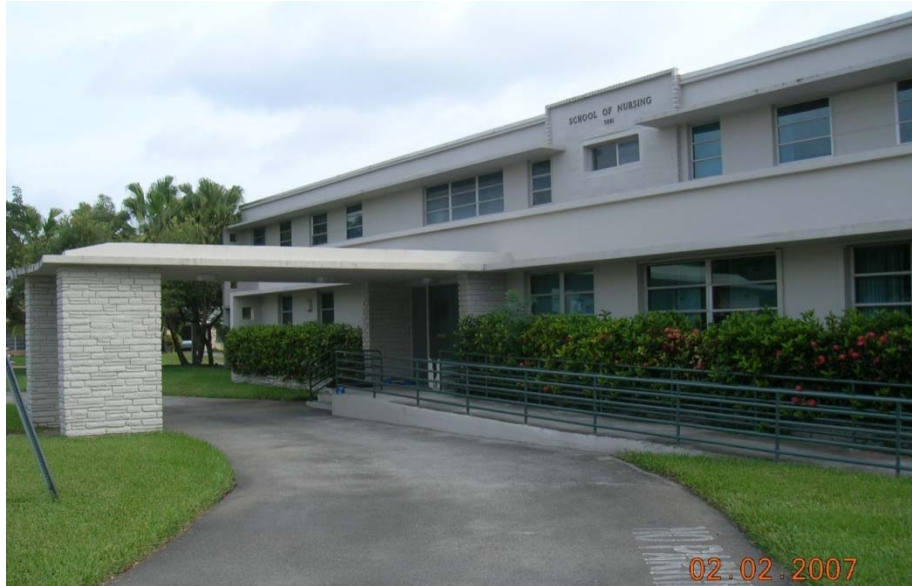
Figure 35 – Test Site: School of Nursing Building
