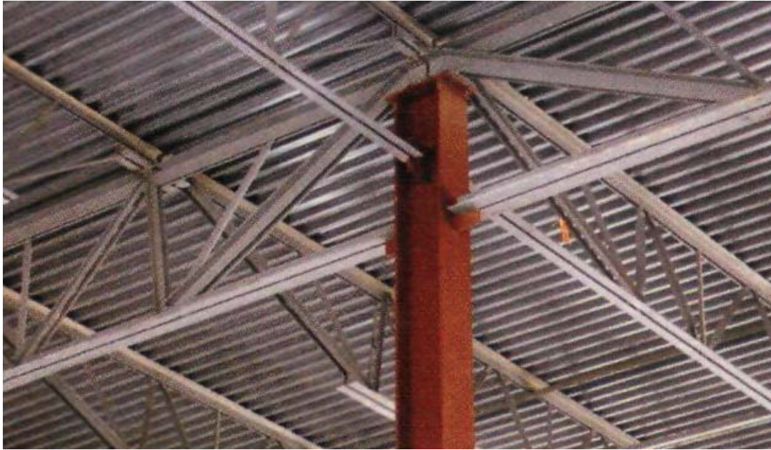
Figure 5 – Steel Joist – Column Connection (Hopleys, 2006)
