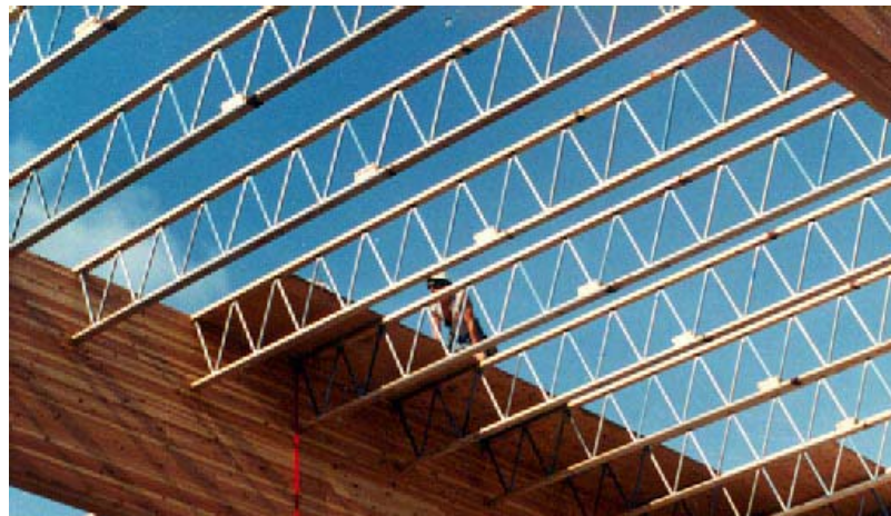
Figure 4 - Light-Weight Floor System (Hopleys, 2006)
