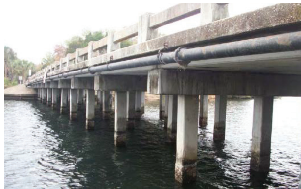
Figure 54 - Existing bridge over the Halls River
