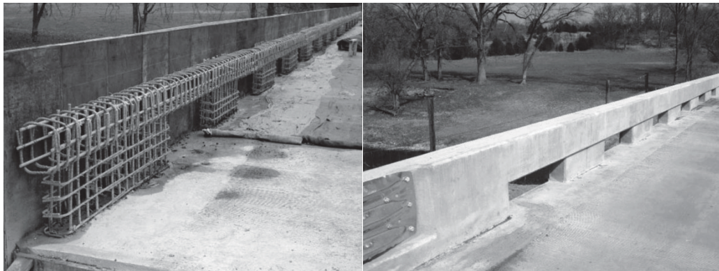
Figure 3.4 - Reconstruction of Bridge No. 14802301 (a) GFRP reinforcement cages prior to casting of railing, (b) open-post railing in service.
