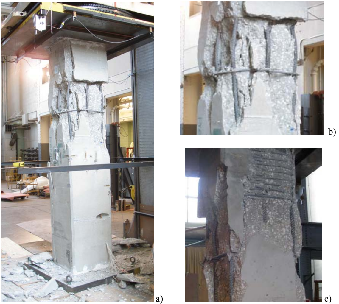
Fig. A - 22: Failure of Specimen S-1-control (a-c).
