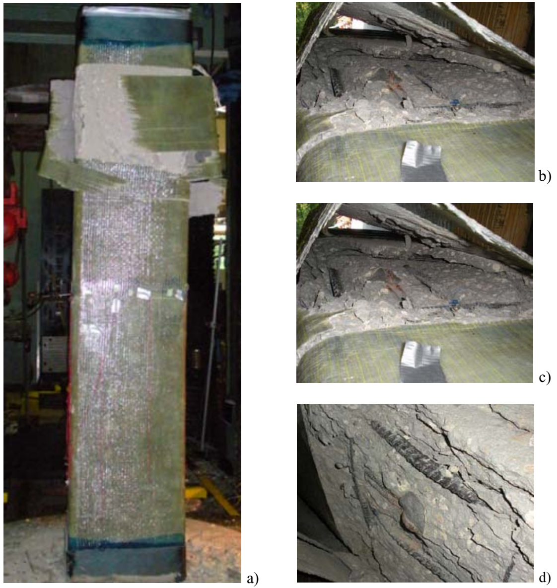
Fig. A - 24: Failure of Specimen S-1-2GB (a-d).
