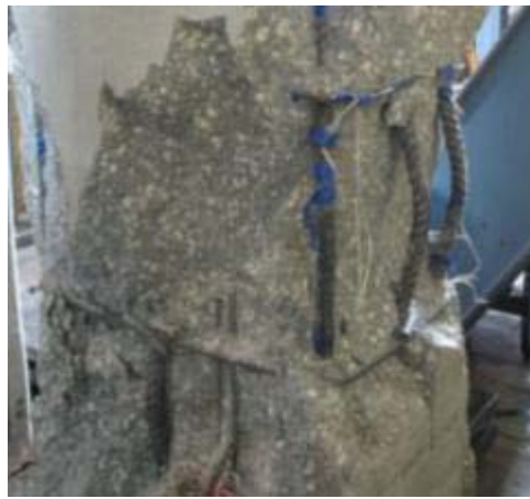
Fig. A - 26: Failure of Specimen R-1-control (a-b).
