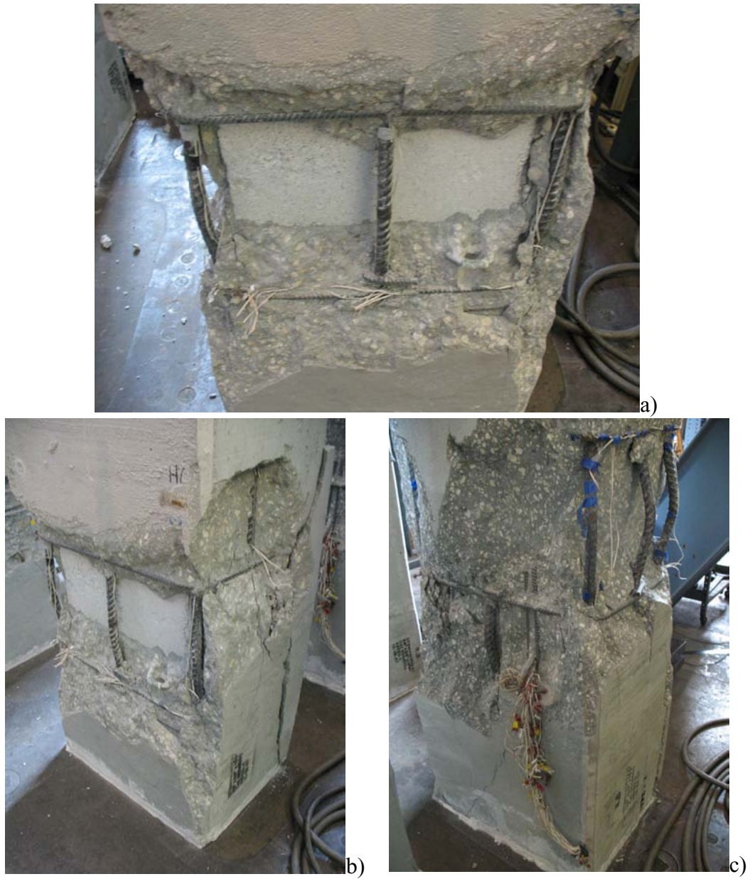
Fig. A - 39: Photographs of failed Specimen HR-control (a-c).
