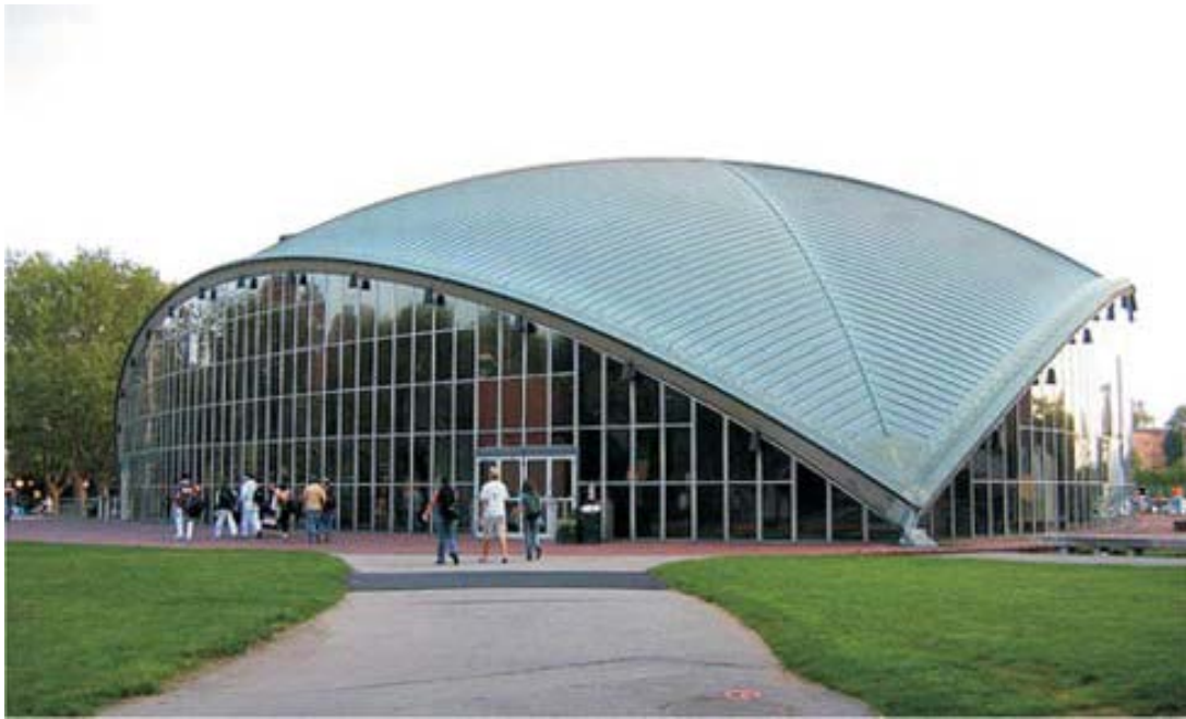
Figure 2.6. Kresge-MIT Auditorium, Boston, USA [13]
