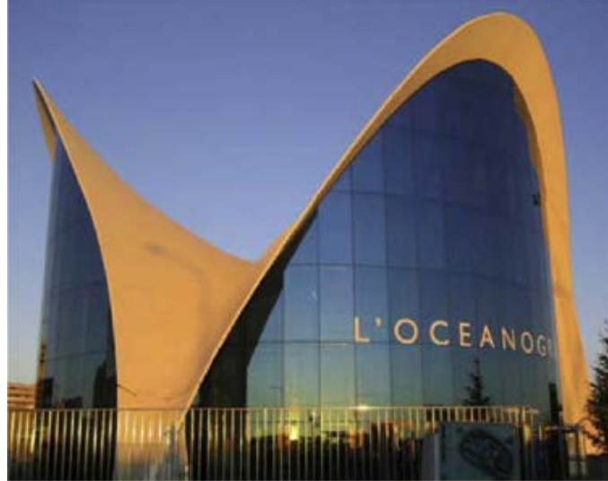
Figure 2.8. Hypar shell structure at the entrance of the Universal Oceanographic Park (Valencia, Spain) [23]
