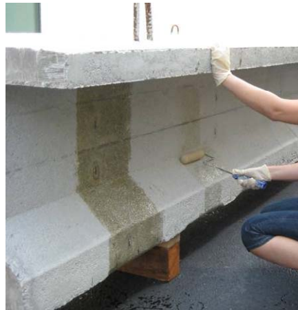
Figure 5.1 – Application of Primer Figure 5.2 – Application of Putty
