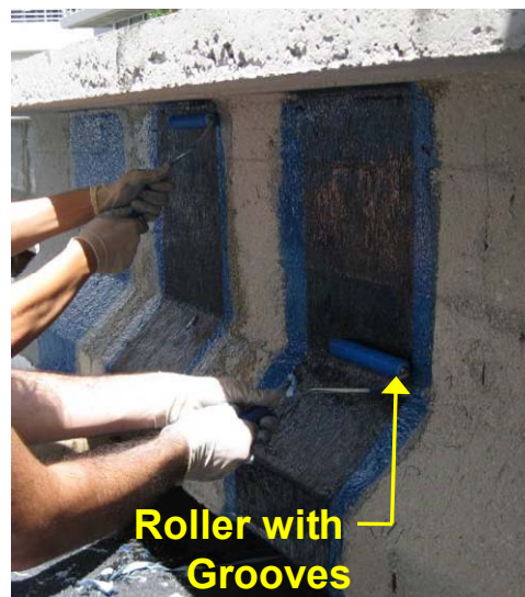
Figure 5.4 – Application of Sheet Figure 5.5 – Removal of Air Voids
