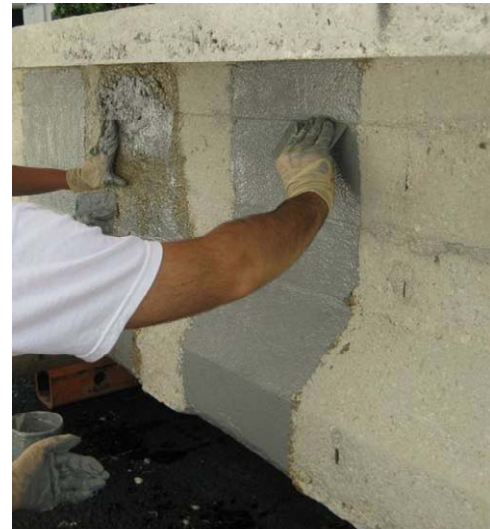
Figure 5.1 – Application of Primer Figure 5.2 – Application of Putty
