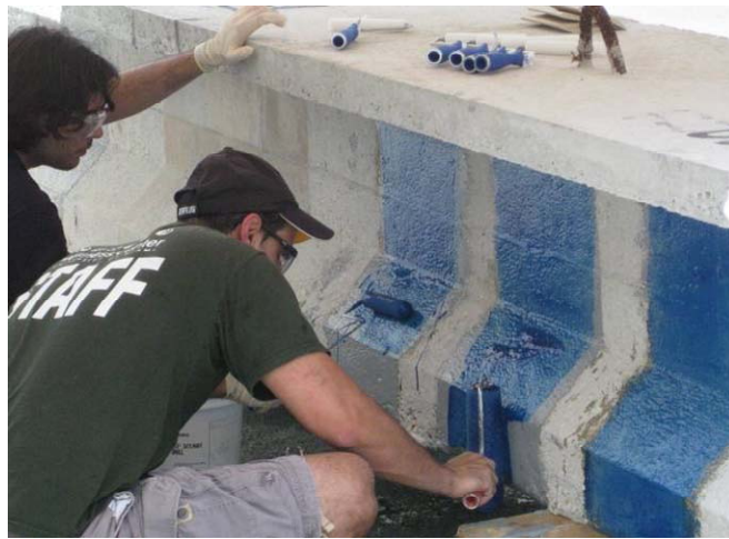
Figure 5.3 – Application of Saturant
