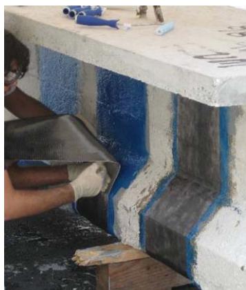
Figure 5.4 – Application of Sheet Figure 5.5 – Removal of Air Voids
