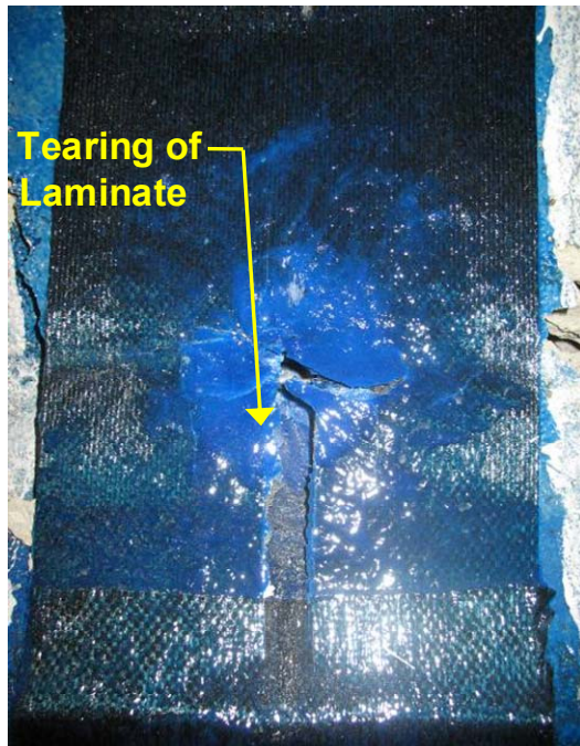
Figure 7.35 – B-4a Failed Laminate
