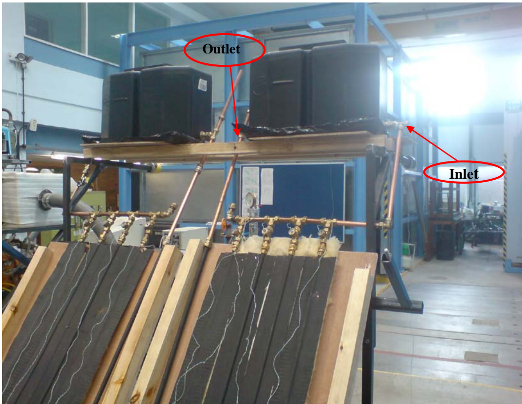
Figure 6.4b Water tanks connected to the collectors.
