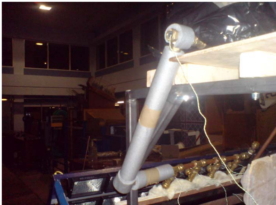
Figure 6.4c Insulated water tanks and copper pipes.
