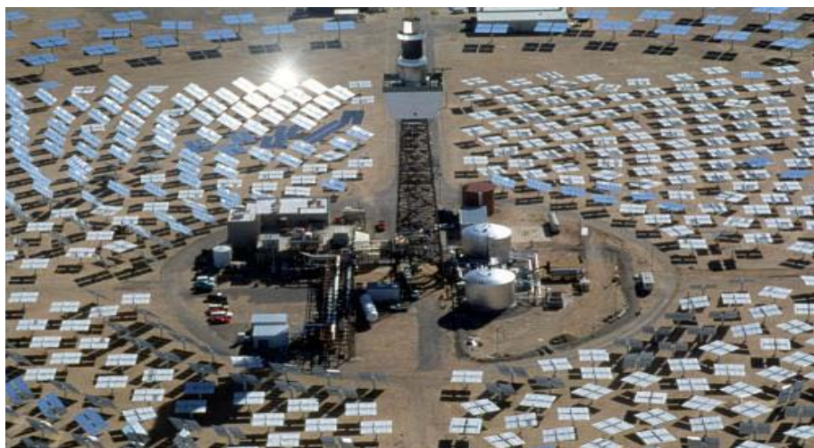
Figure 2.6a A Central Receiver System [13].
