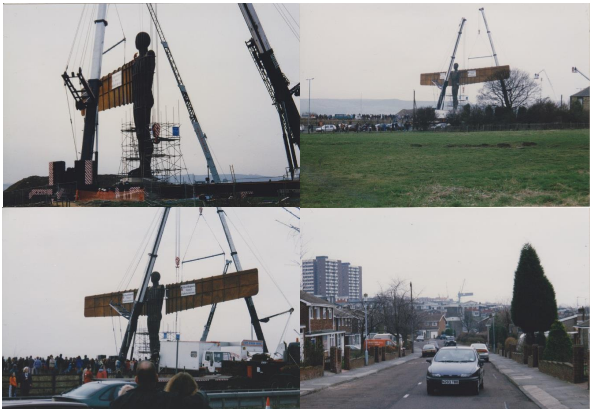
Figure 4.3: The Angel in construction. Images courtesy of Alan Ford
