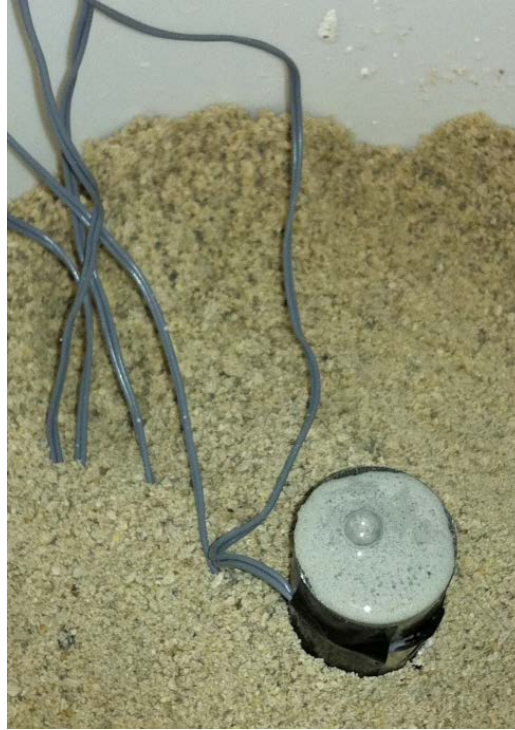
Figure 8 Pipe filled with grout
