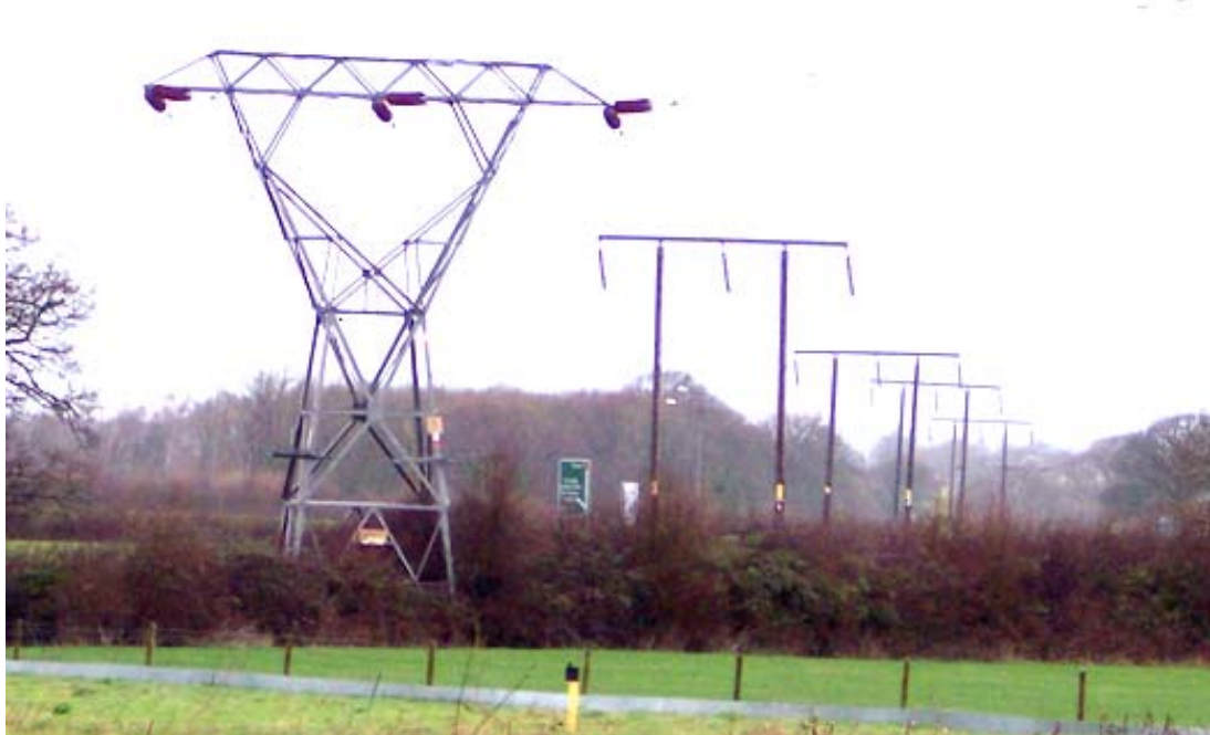
Fig. 7.5 A part of SPEN network (7 km) OHL 132 kV from Rhyl to St.Asaph on north east coast of Wales
