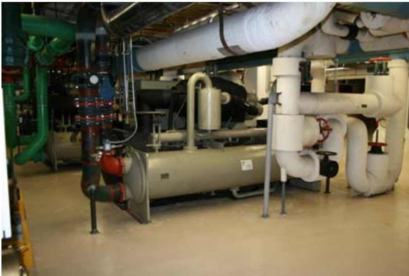
Figure 3-3 200-ton screw chiller.
