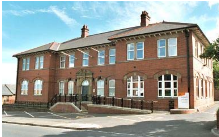
Figure 6.12: Building Ten: EDC ‘Main Building’
