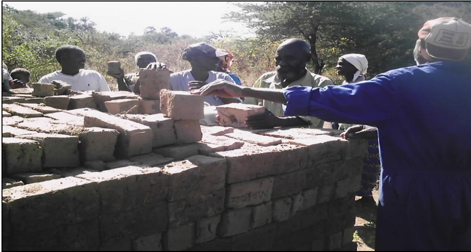
Figure 5 Community members making bricks for the construction of public toilets
