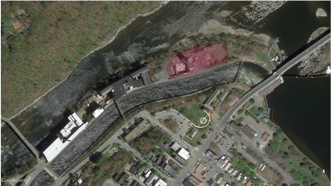
Figure 17: Aerial view of the Power Island
