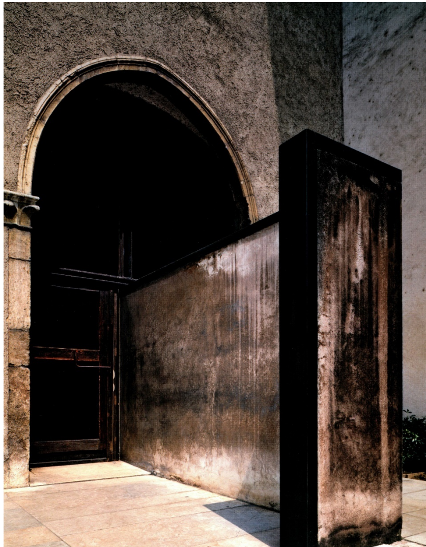
Figure 2: A concrete form protrudes out of the historic space to mark the entrance into the Castelvecchio
