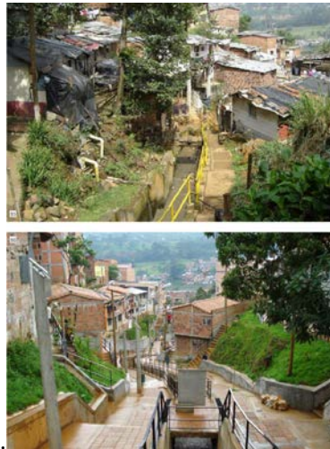
Figure 32: PUI circulation, runoff, and green infrastructure upgrade
