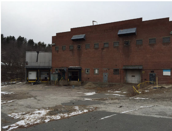
Figure 26: Pellet Production Plant. Image by author
