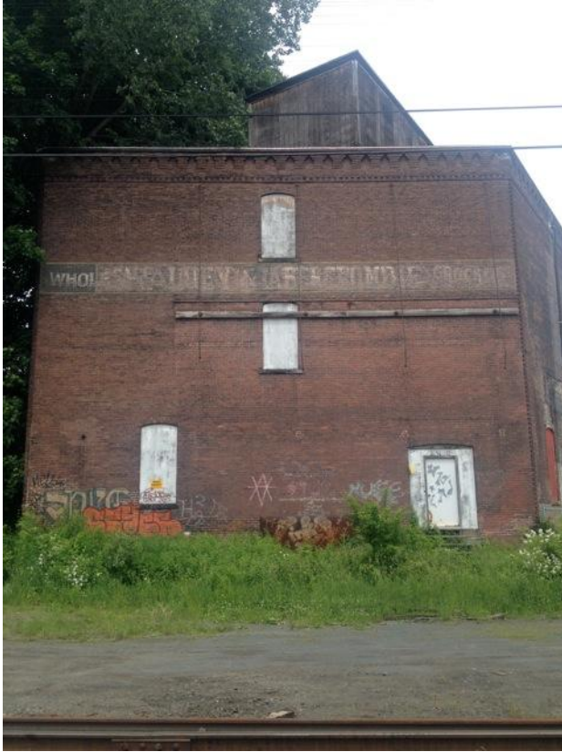
Figure 14: The West facade
