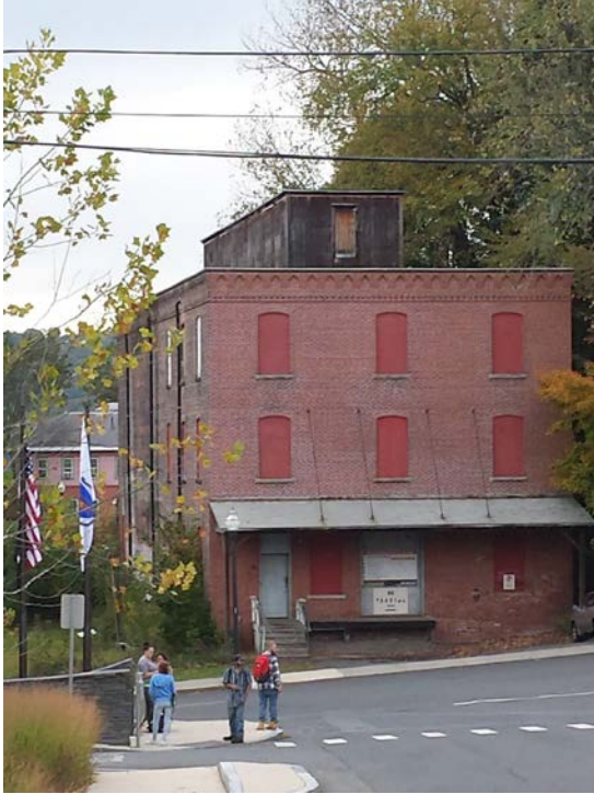
Figure 12: Existing front (East) facade
