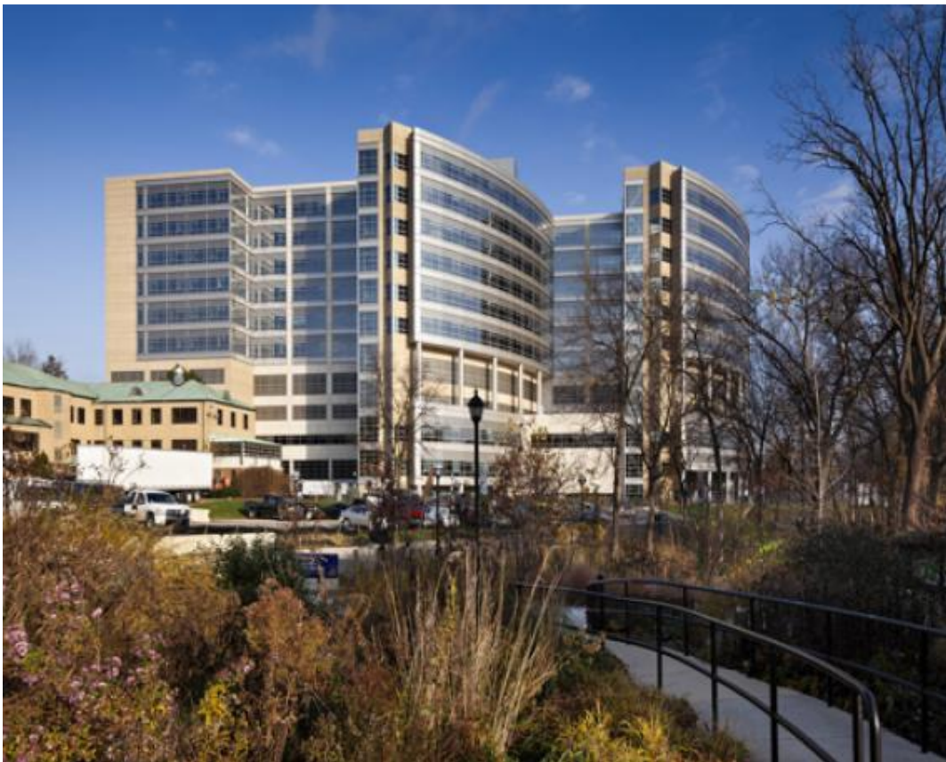
Figure 22. Facade Glazing (Image credit: CS Mott Children's Hospital Website)
