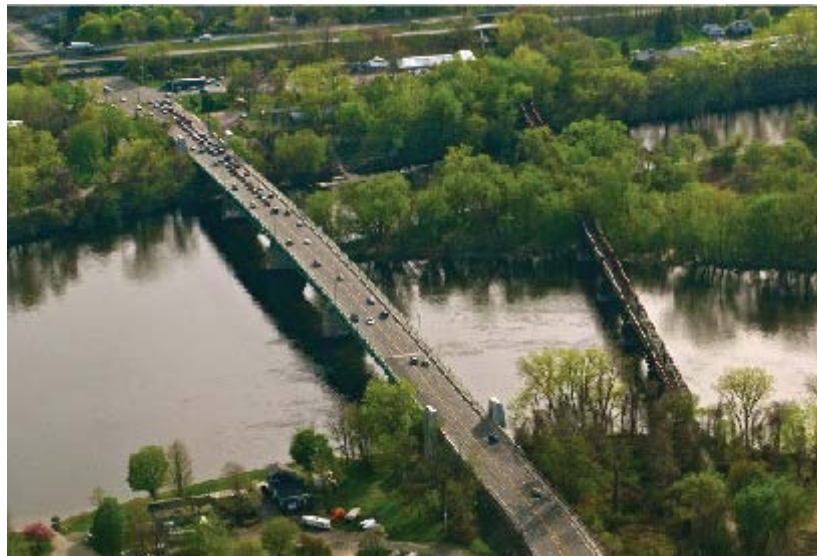
Figure 14- Calvin Coolidge Bridge on the left and Norwuttok Rail Trail Bridge on the right
