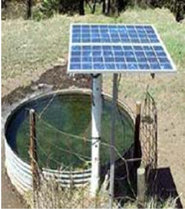
Fig. (3.17) PV water pump in one of the Palestinian villages
