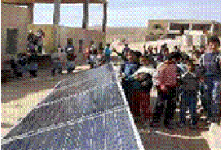
Fig. (3.18) School PV system in one of Palestinian's villages
