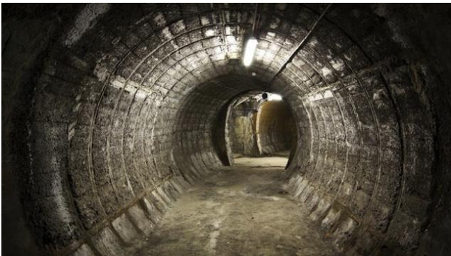
Figure 2: Abandoned underground track
