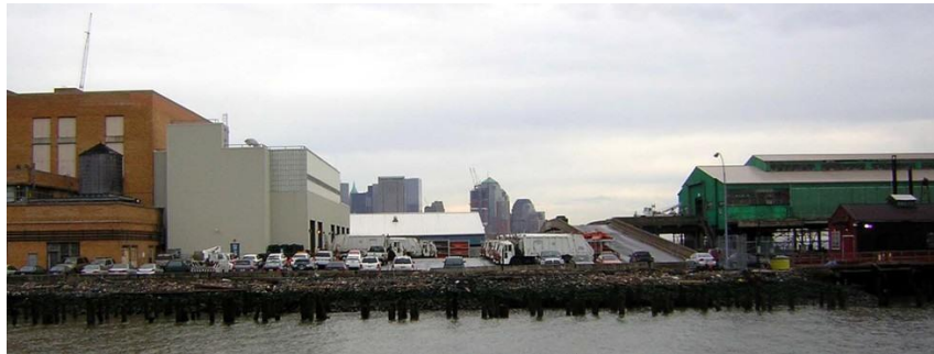
Figure 34: View of Gansevoort Peninsula from Hudson river
