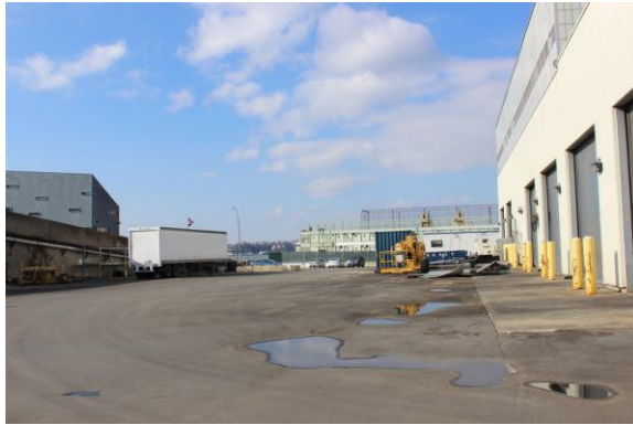
Figure 33: View of Pier 53
