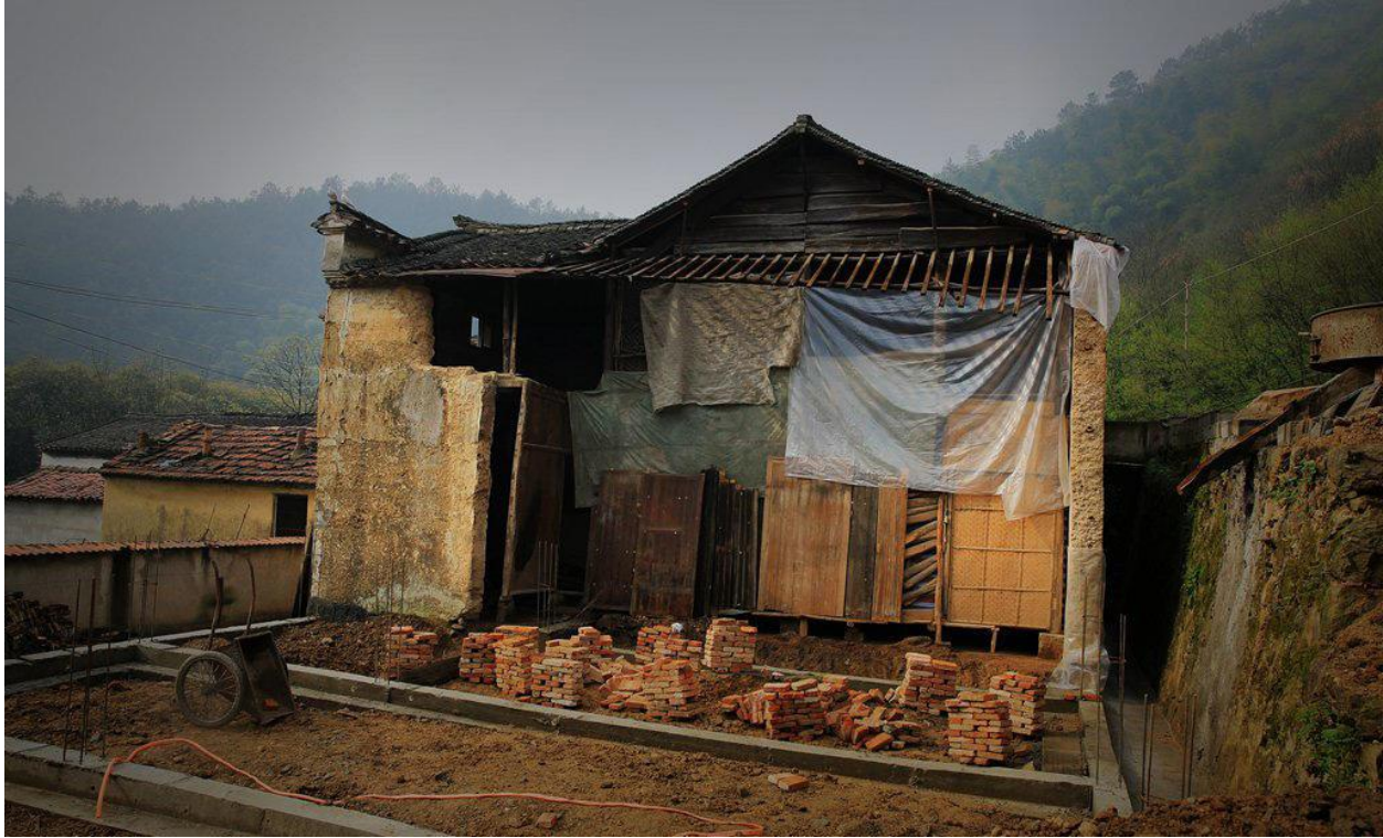
Figure 25 The house of Dasan Cao which are under demolition
