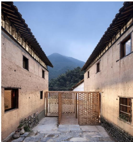
Figure 60 The addition connects the existing two
