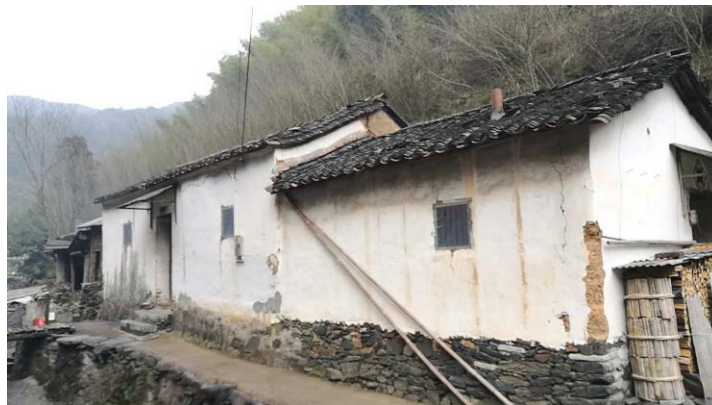
Figure 35 Three buildings connected as one house in Xiawan
