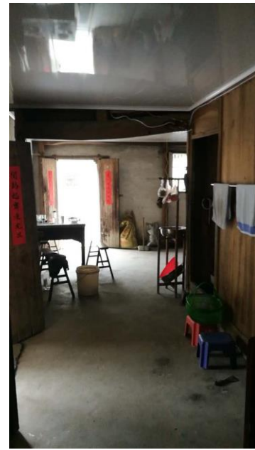
Figure 76 Existing interior view
