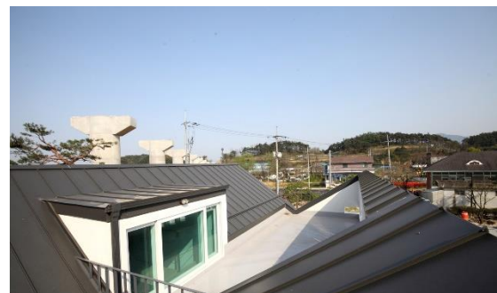
Figure 47 Roof view of the house
