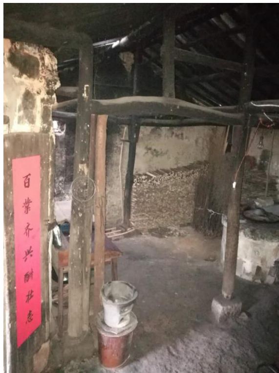
Figure 78 Existing interior view
