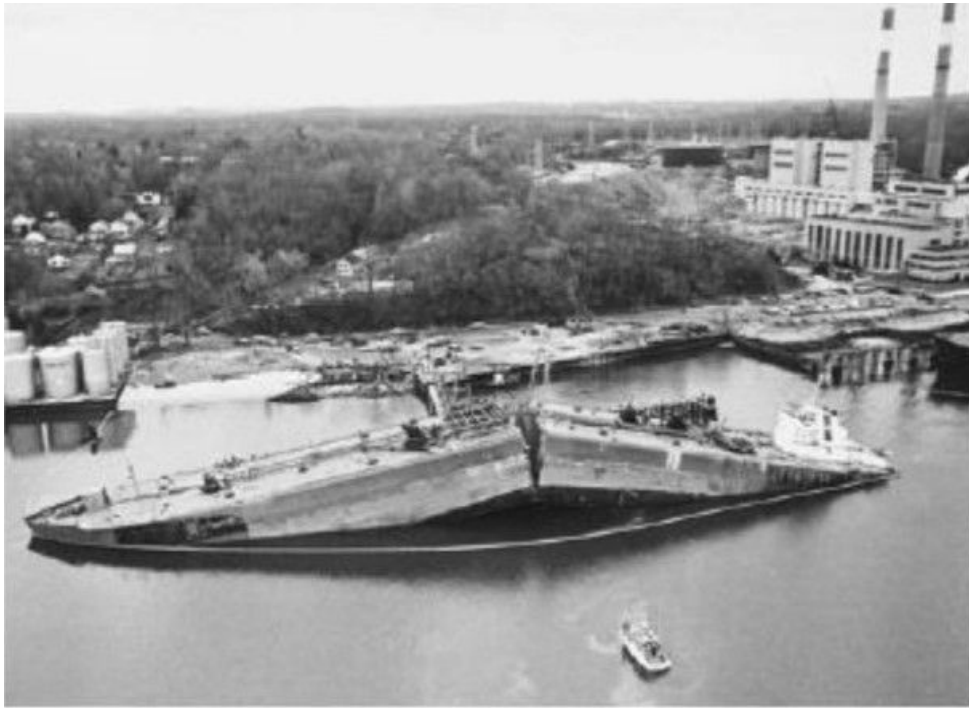
Fig. 1.1. Fractured Liberty ship located at dock. Extracted from [6].
