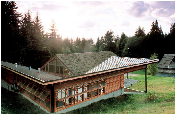
Figure 18 – Pilchuck Glass School - Studio Annex.
