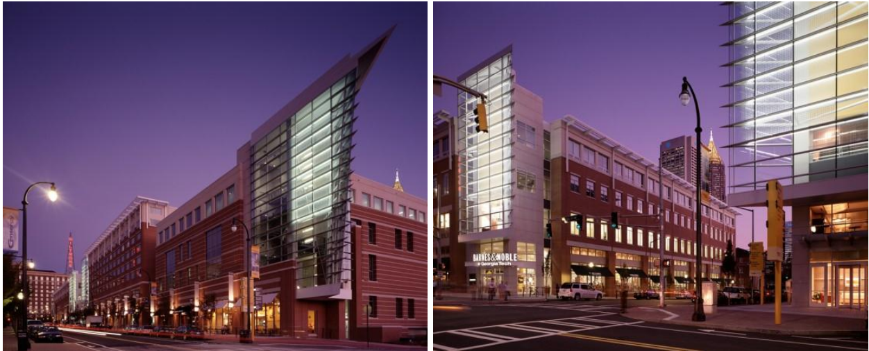
Figure 4-30. Landmark architecture of Technology Square, Atlanta. Source: TVS Design (2011). Retrieved May 21, 2011, from http://tvs-design.com/
