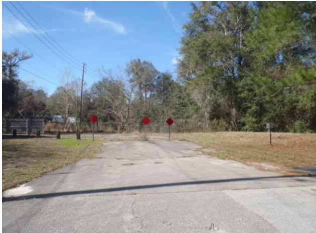
Figure 4-21. Image of Linton Oaks discontinued SW 8 th Avenue (Amanda Douglas, 2013)
