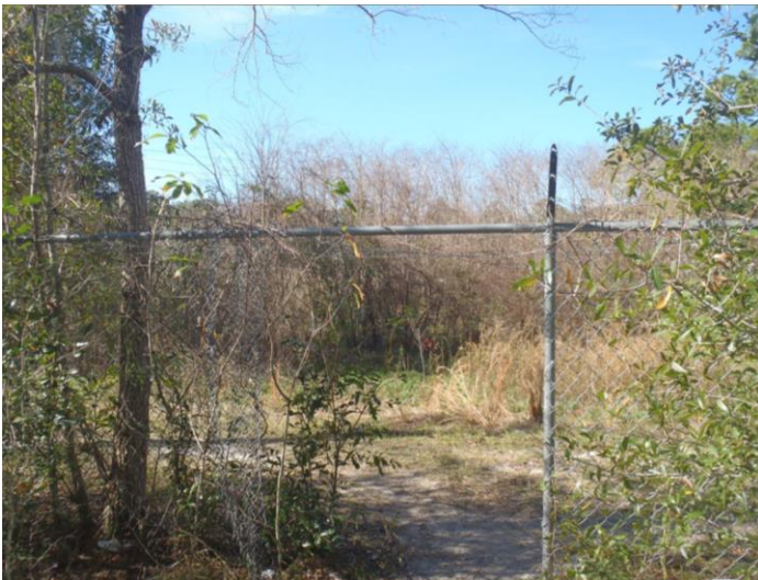
Figure 4-15. Linton Oaks SW 8 th Avenue informal path leading to damaged fence and trespassing (Amanda Douglas, 2013)
